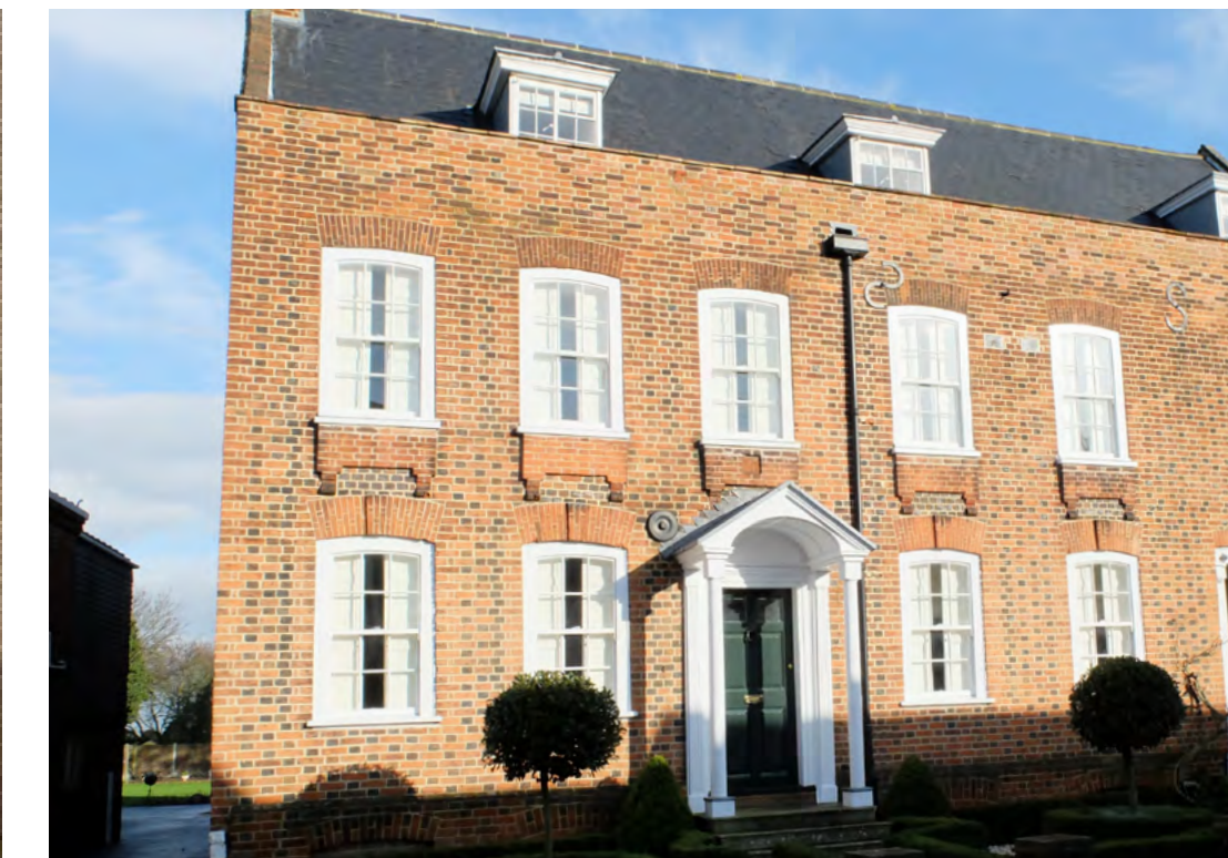
Figure 128. Materials to reflect a domestic character within the residential areas. Horndon on the Hill
