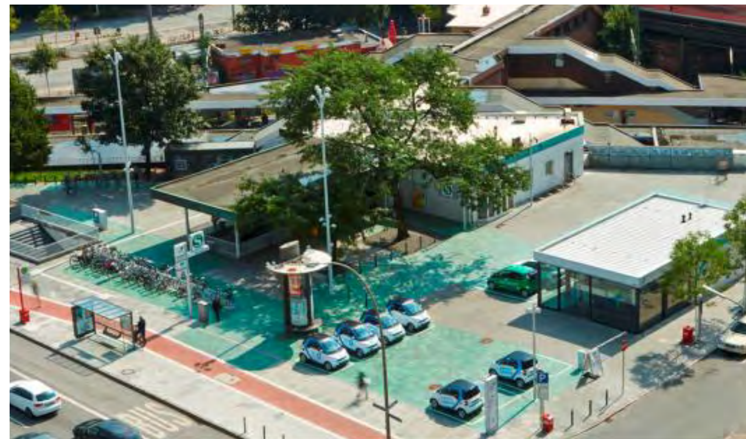
Figure 113. Mobility hub with a range of services ranging from travel planning to physical infrastructure
