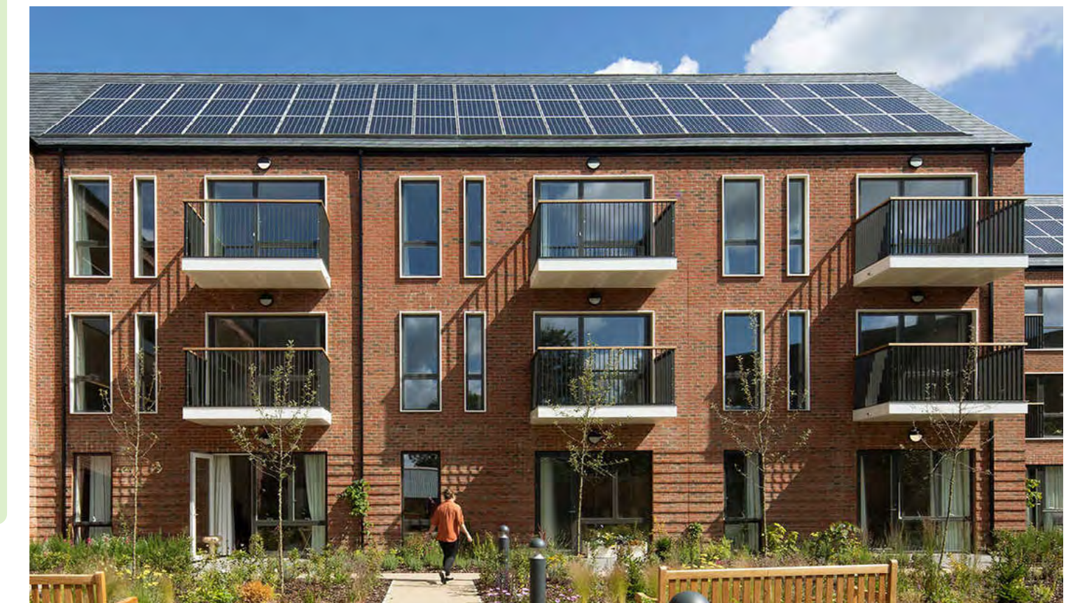
Figure 124. Larger openings to capture long views within Dunton Fanns, Ansell Court, London. PRP Architects.
