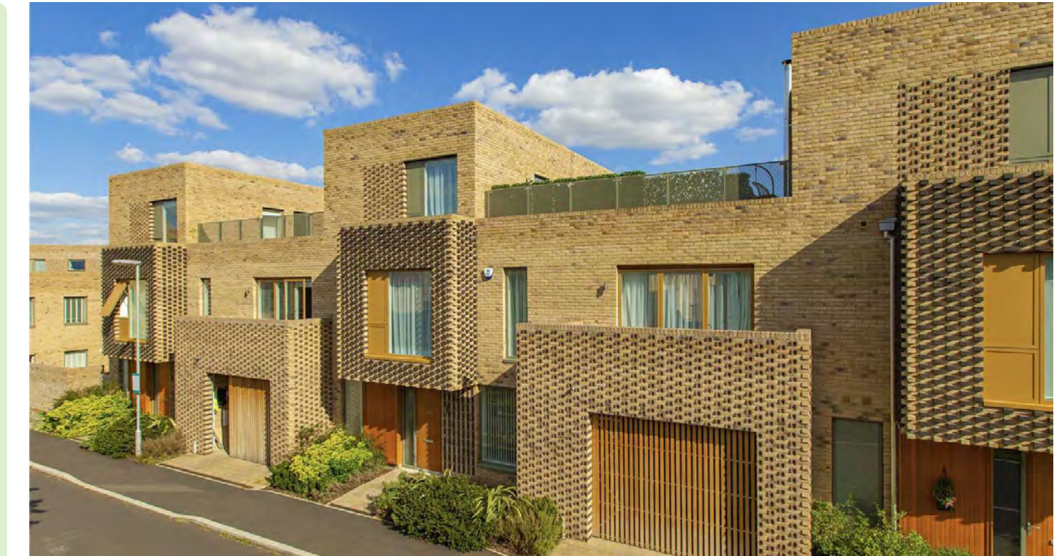
Figure 123. Extrusion of elements combined with material change can create visual interested and provide a varied roof-line expression. Hobson Road, Trumpington, Cambridge
