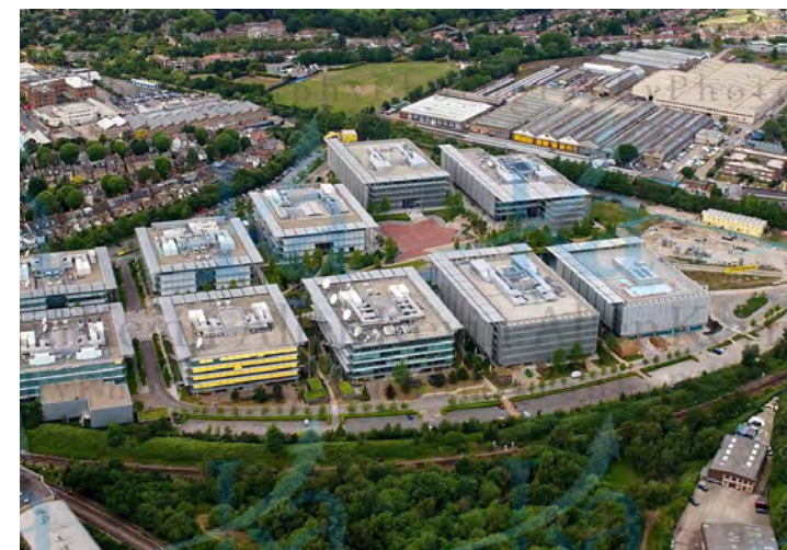
Figure 133. Consistency in design across all the buildings. ake/ Grow Alconbury Weald - AHMM Architects
