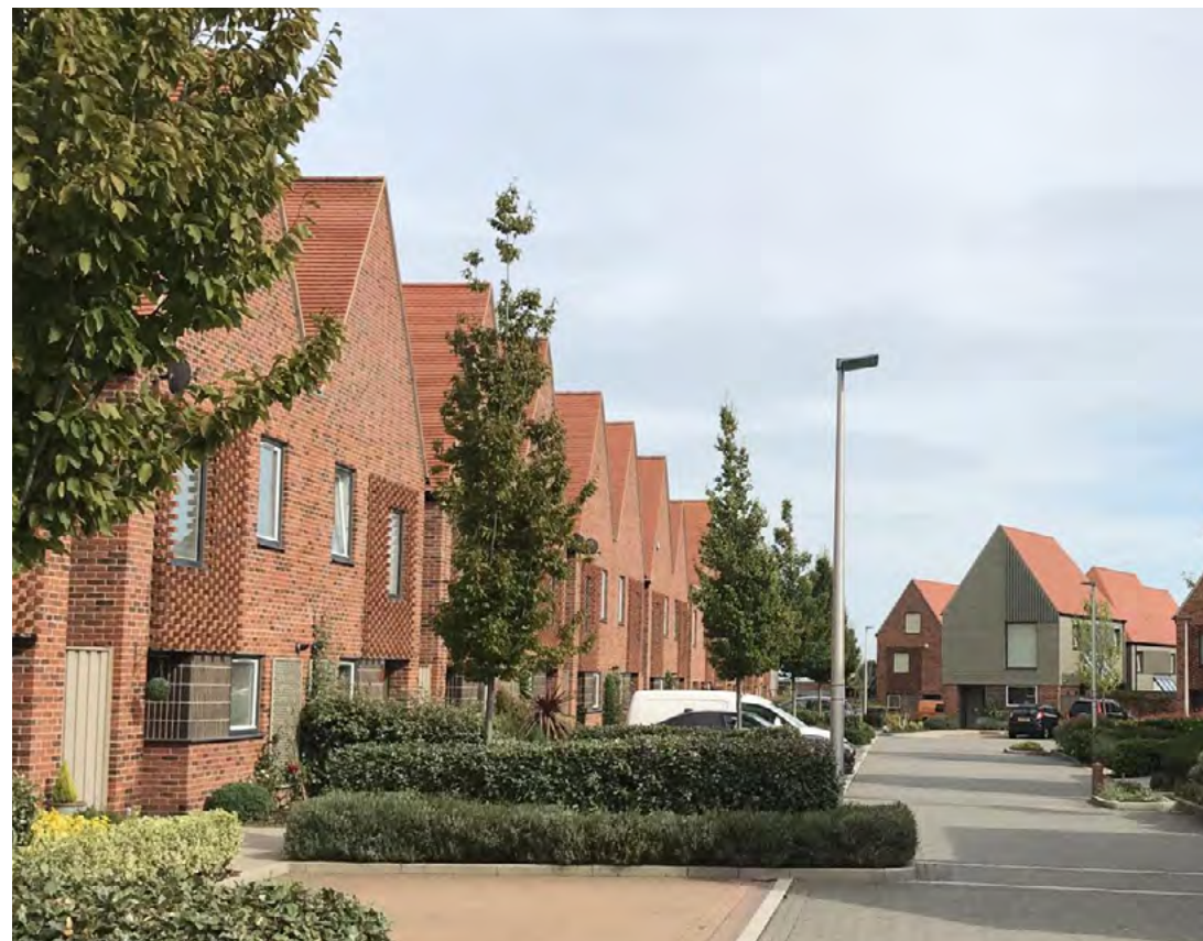
Diagram 53. Continuous roofing along a continous building line. Horsted Park, Kent - Proctor & Matthews
