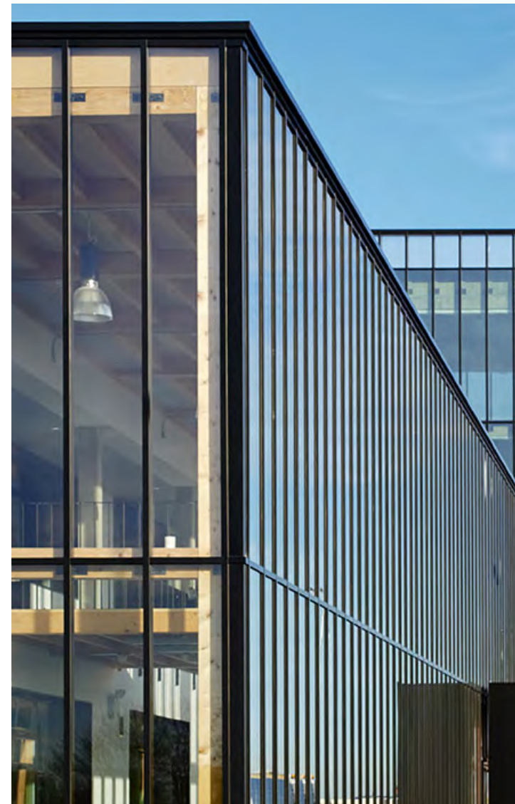
Figure 131. Emphasis on verticality with the use of curtain walls. Alconbury Incubator - AHMM Architects
