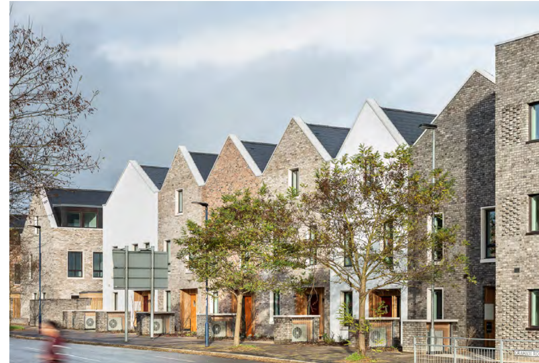
Diagram 52. Gables creating a stronger presence along the streetscape. Marmalade Lane, Cambridge - Mole Architects
