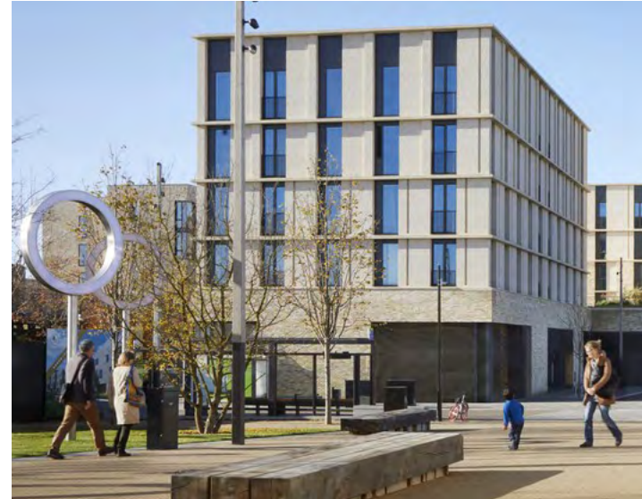
Figure 130. Large windows that maximise internal light. North-west Cambridge Business Park - Stanton Williams Architects
