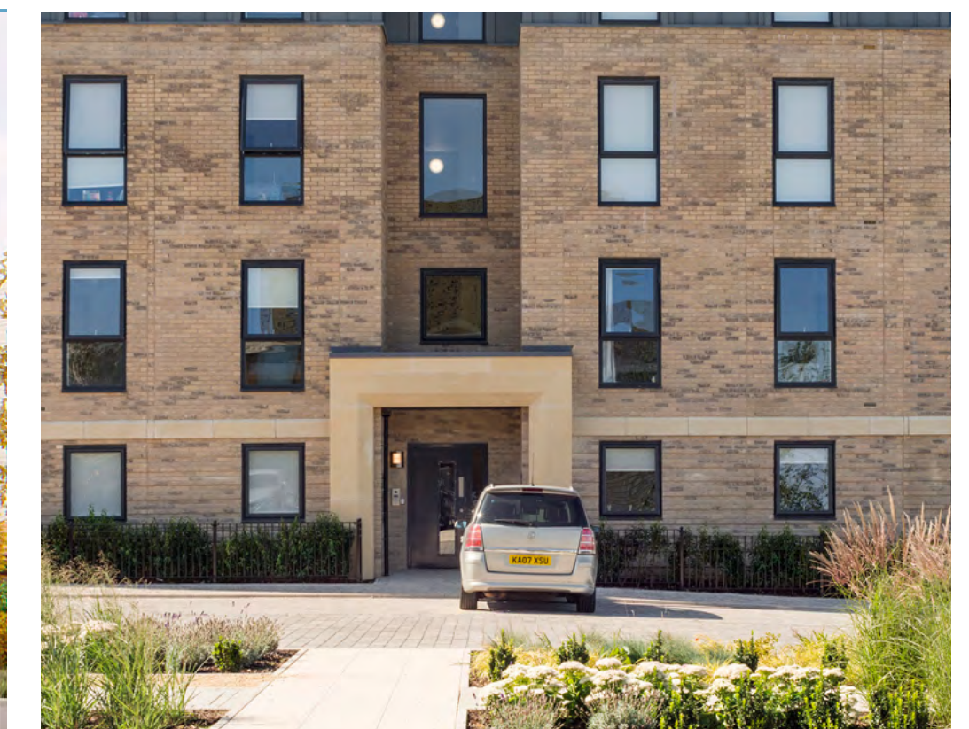
Figure 120. Use of varied material to emphasize on entrance to apartments. Mulberry Park, Bath - HTA Design
